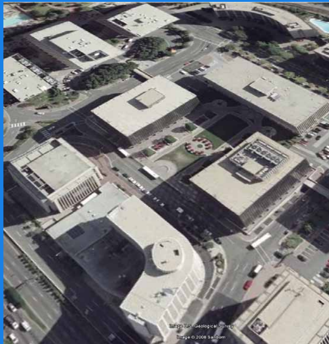
Existing block between 20 th and 18 th Streets
